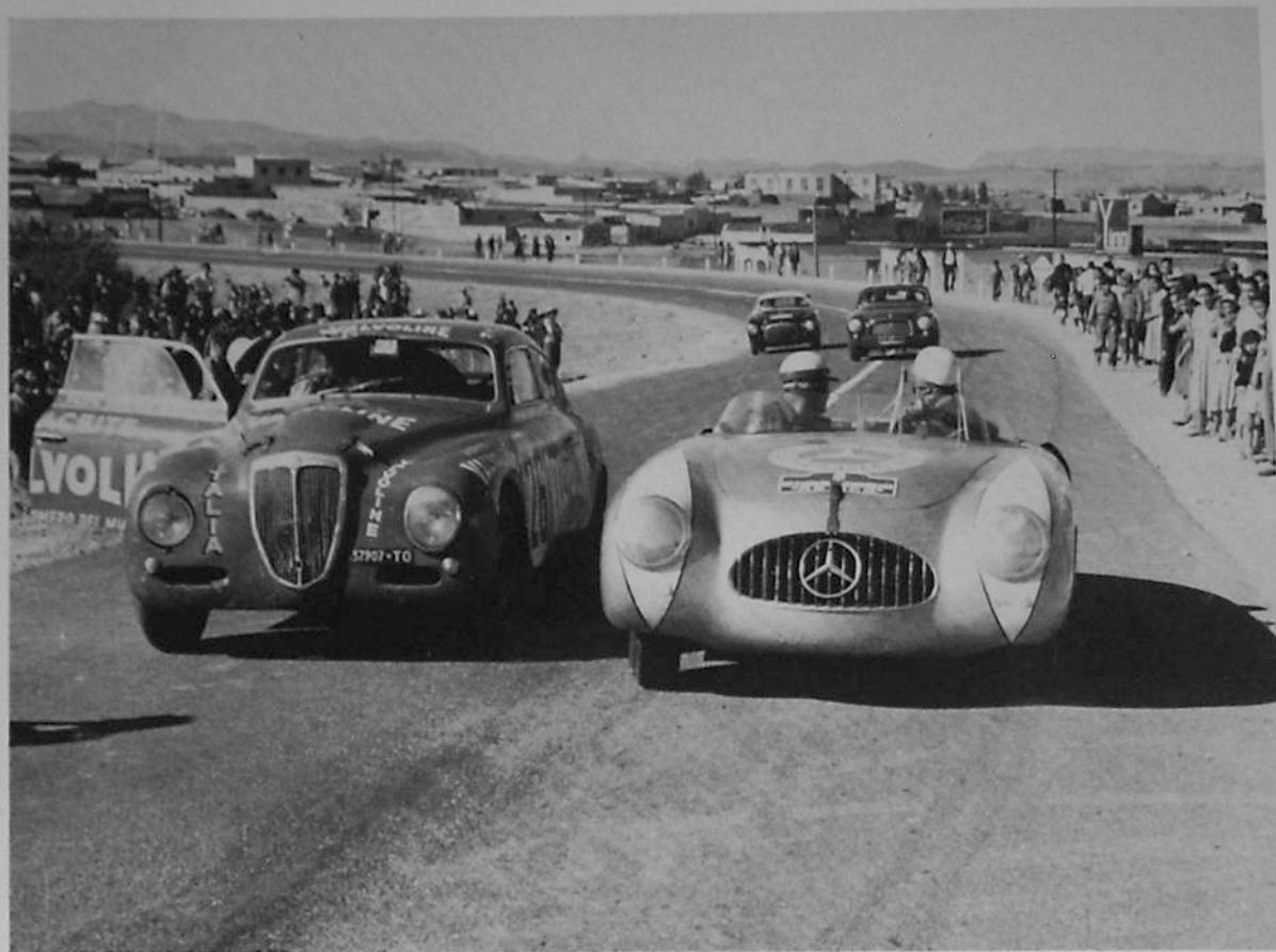
1952 Carrera Messicana. The Lancia Aurelia B 20 special with lowered aluminum body and Roots compressor, driven by Umberto Maglioli, prepares to start a leg. On the right, the Mercedes 300 SL of American John Fitch, who in that moment had shifted into reverse to return to the pits for a small repair. He was later disqualified for driving "against the race direction". Mercedes later commented: "A problem between North Americans and Mexicans..."
